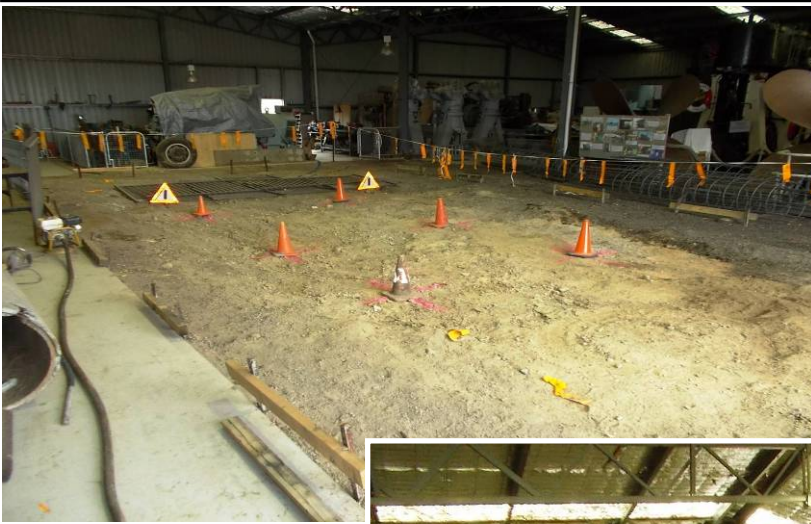
Left Bay 4 with hurdles and string lines marking out the foundation extremities and pier locations.
