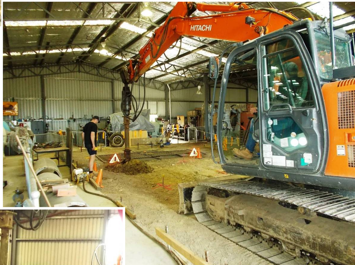
Below Starting the first hole . The boring rig fits on the end of the excavator boom and is driven through a square drive fitted to a geared hydraulic motor which is controlled and computer monitored from the cabin .
