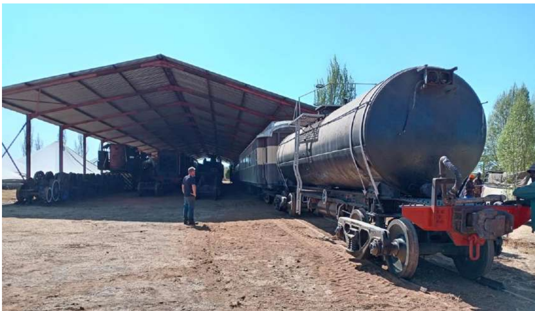
After additional track was laid at the end of the shed, the water tankers were rolled out and the coaches placed in front of them by crane and then rolled back under the shed.
