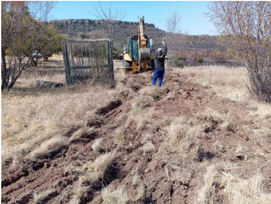
Building a road out of the Ladybrand site.
