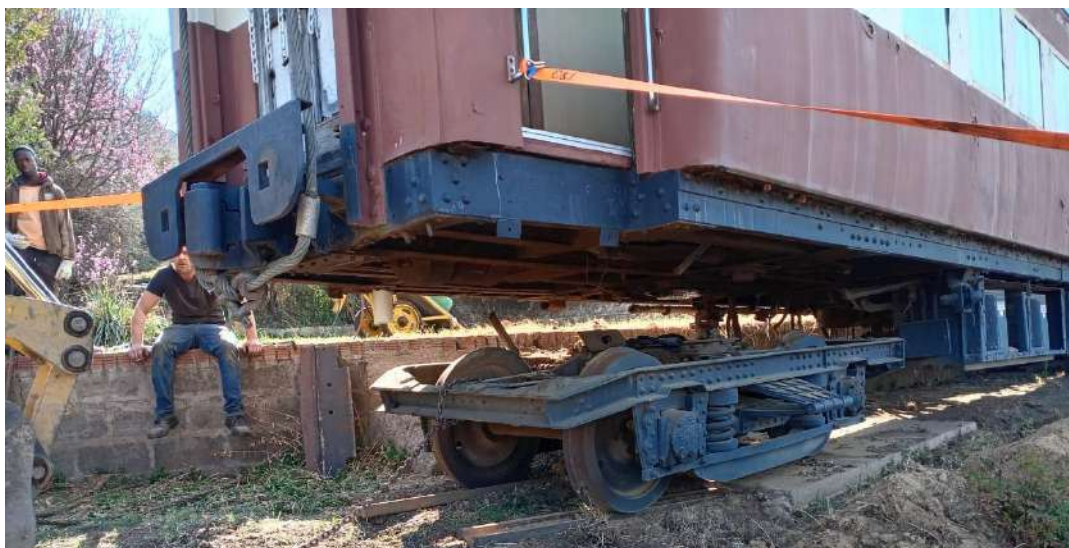
Removal of the rail bogie.
