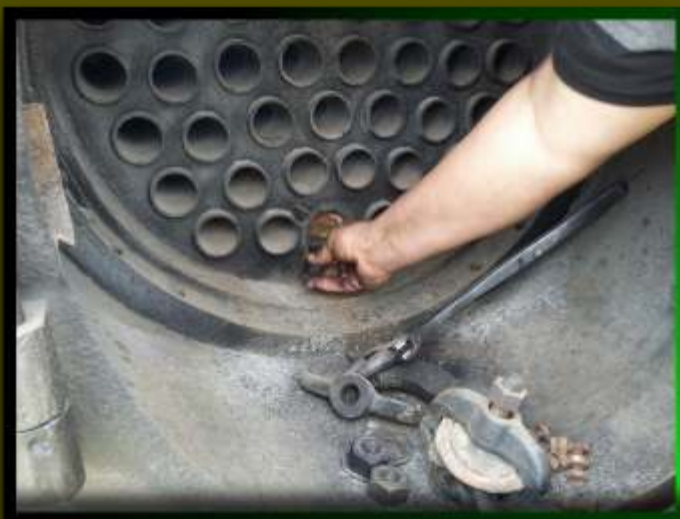
Below right: Cleaning all soot from the tubes with a tube cleaner.
