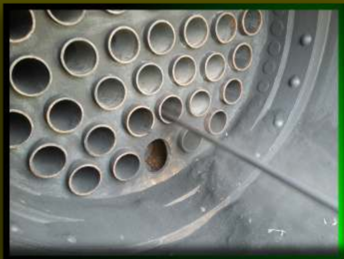
Below right: Cleaning all soot from the tubes with a tube cleaner.
