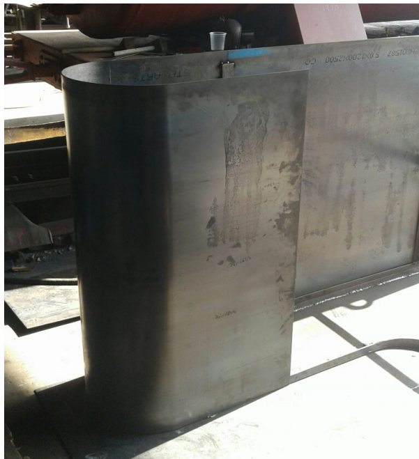
The first plating has been rolled for the coal bunker. Picture by Lukas Nel.
