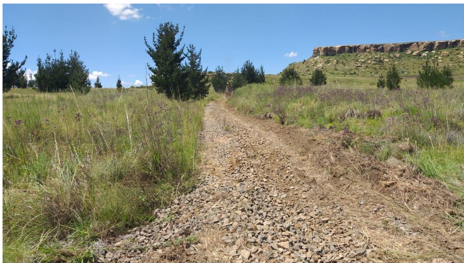
The first track panels of the mountain section are being lifted.
