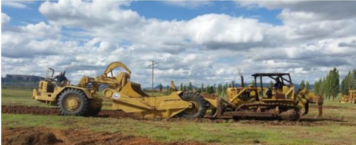
Dig it! An earthmoving demonstration in 2019.
