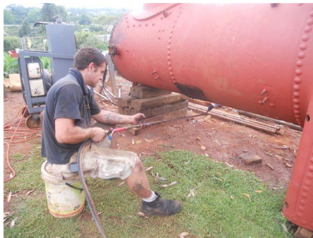
Heating the area prior to the pressing out of the bulge
