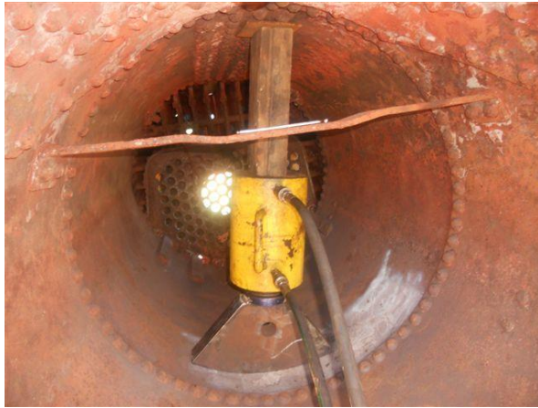
Pressing out the bulge in the boiler barrel
