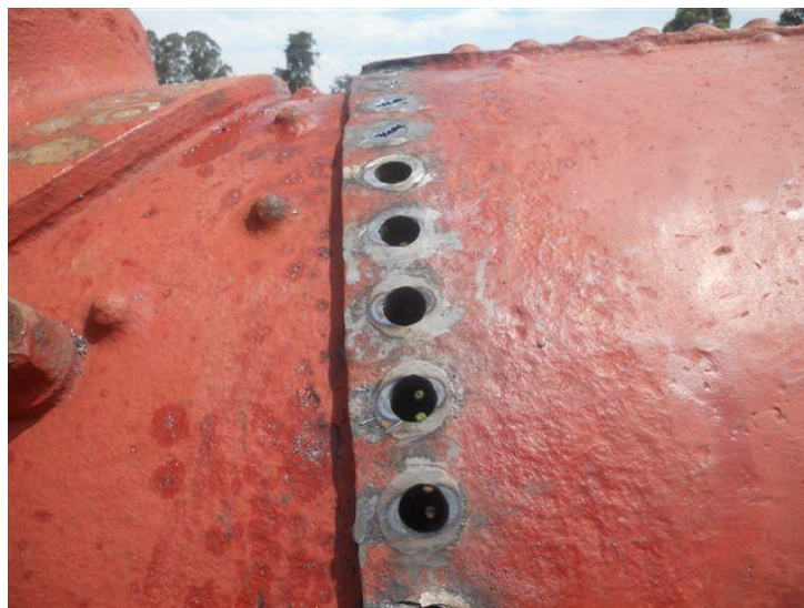
Rivets removed
