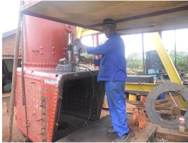
The throat plate stays being drilled out
