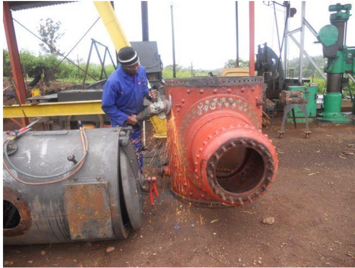
Stripping the dome section
