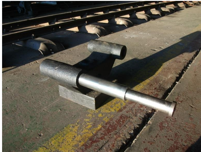
The refurbished front bogie center.
