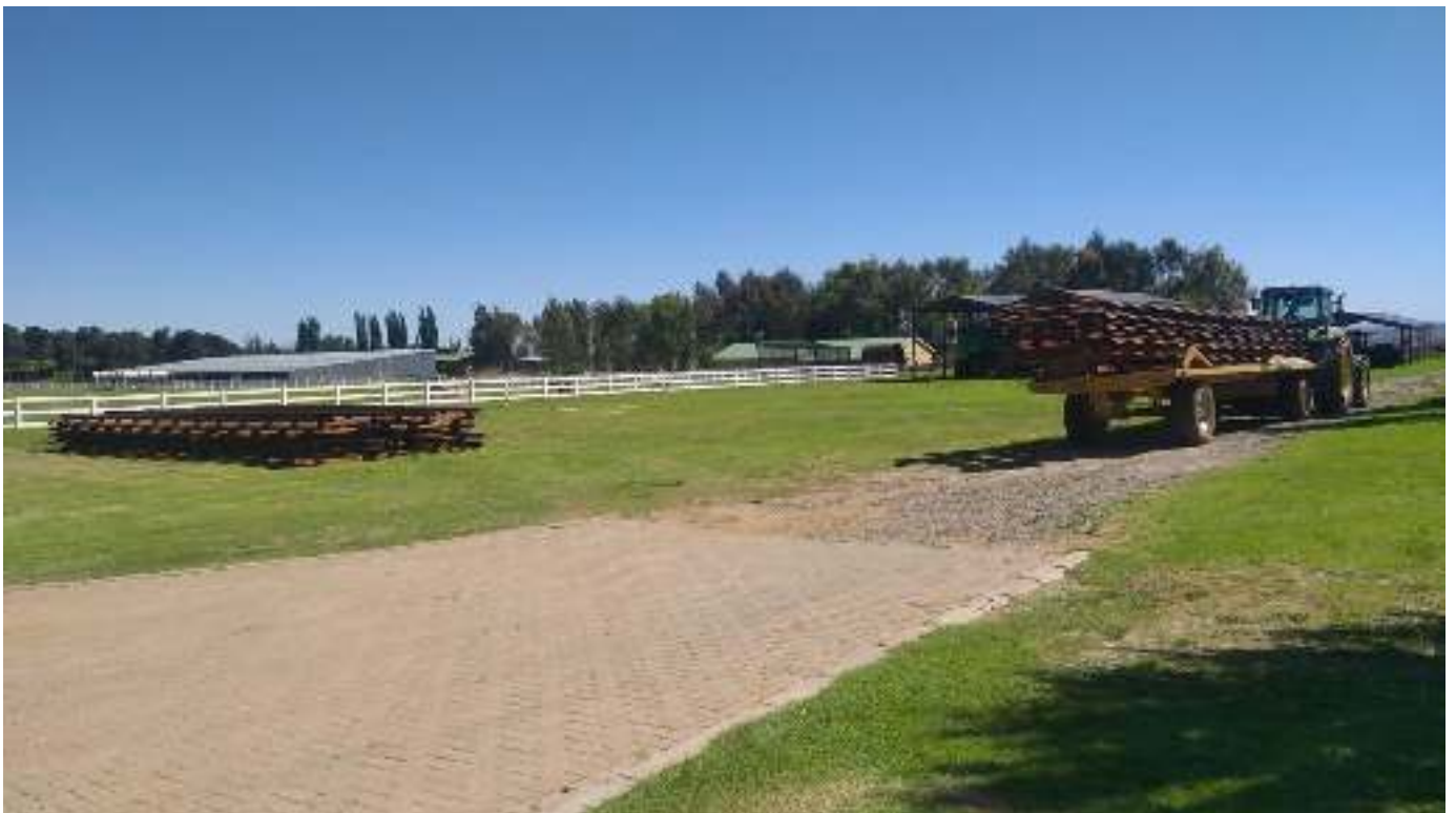
Newly fabricated 3' 6" gauge track panels are brought on to the display site for the impending arrivals. Picture by Sandstone Heritage Trust.
