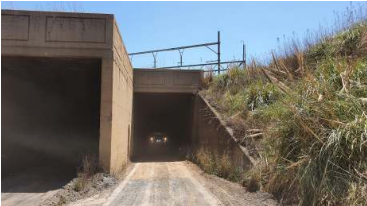
The bottleneck at Germiston, the limited clearance exit tunnels. Picture by Shaun Ackerman, Fairlie Projects.
