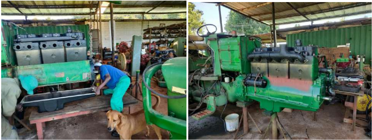
Fitting the sump and on the right the sump pan in place.
