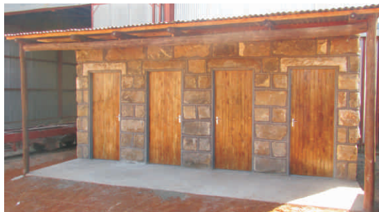
Below: The new Sleeping Coaches Ablution Block situated at the end of the carriage shed
