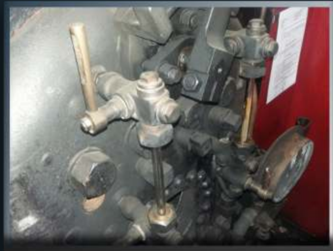
Below left: Old gauge glass being removed.
