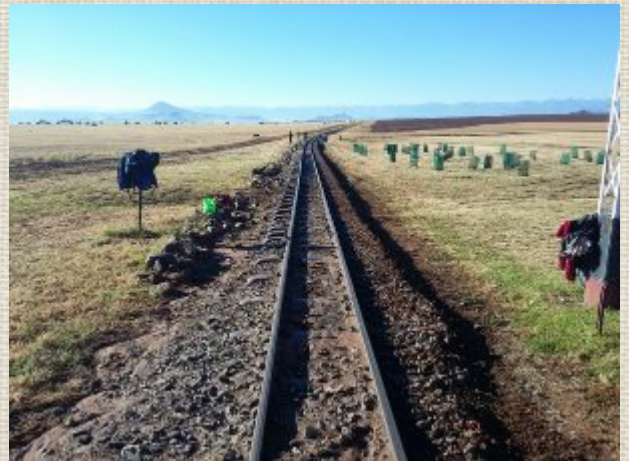
This week we started with our track maintenance and first boxed the ballast opposite the Hoekfontein Station South gate.
