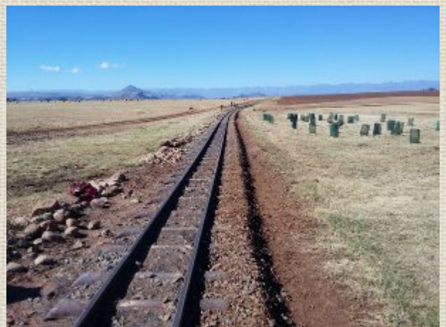
This week we started with our track maintenance and first boxed the ballast opposite the Hoekfontein Station South gate.
