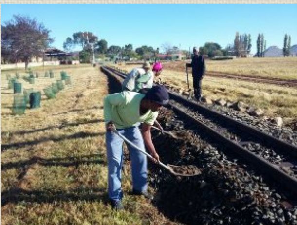
This week we started with our track maintenance and first boxed the ballast opposite the Hoekfontein Station South gate.
