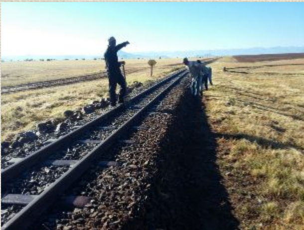
This week we started with our track maintenance and first boxed the ballast opposite the Hoekfontein Station South gate.
