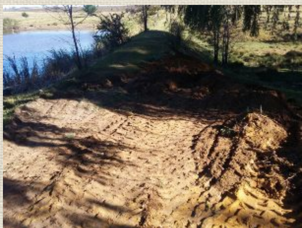
Below: Building up the dam wall with soil from the forest side.
