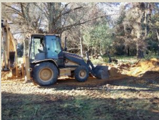
Below right: Thabiso graded the B section a couple of times to get the road smooth and level.
