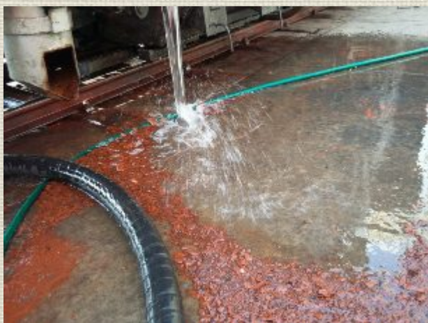
Finally we cleaned the tubes and ensured that no one is blocked with cinders.
