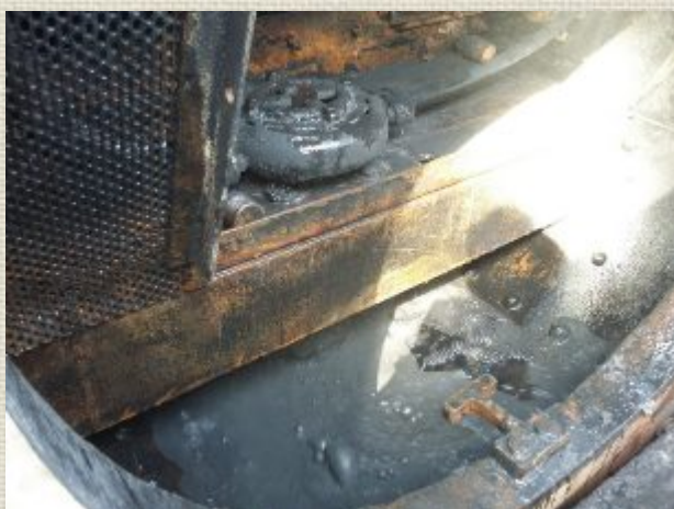
Finally we cleaned the tubes and ensured that no one is blocked with cinders.
