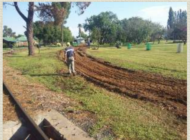
Below: Menasse did all the leveling and worked on a much smoother curve into Hoekfontein Station. The Problem we had is that the short sharp S curves is damaging the NGG 16 steam pipe Ball joints.
