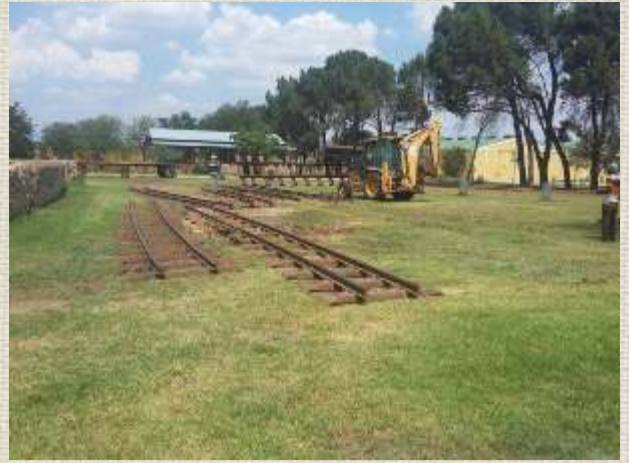
Below right: A much smoother curve than before even though the tightest of this curve is at a radius Of 50 Meter.
