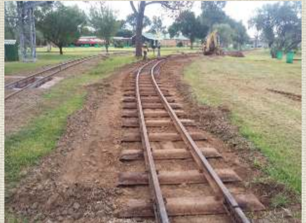
Below right: A much smoother curve than before even though the tightest of this curve is at a radius Of 50 Meter.
