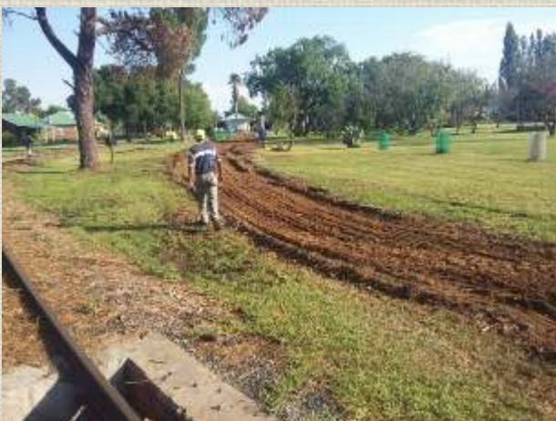
Below: Menasse did all the leveling and worked on a much smoother curve into Hoekfontein Station. The Problem we had is that the short sharp S curves is damaging the NGG 16 steam pipe Ball joints.
