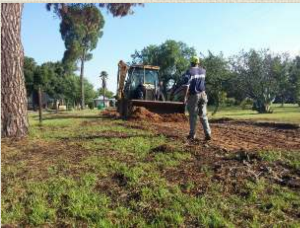
Below: Menasse did all the leveling and worked on a much smoother curve into Hoekfontein Station. The Problem we had is that the short sharp S curves is damaging the NGG 16 steam pipe Ball joints.
