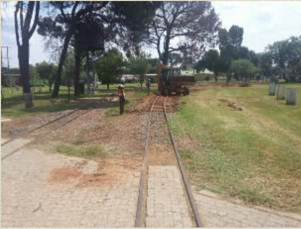
Below right: A much smoother curve than before even though the tightest of this curve is at a radius Of 50 Meter.
