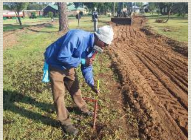
Below: Menasse did all the leveling and worked on a much smoother curve into Hoekfontein Station. The Problem we had is that the short sharp S curves is damaging the NGG 16 steam pipe Ball joints.
