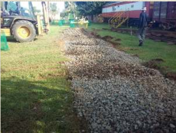
Our Track bed was ready and the 2 panels were fitted.
