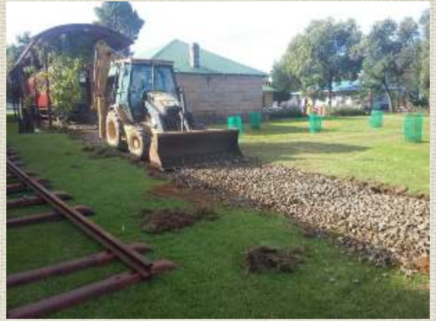
Our Track bed was ready and the 2 panels were fitted.
