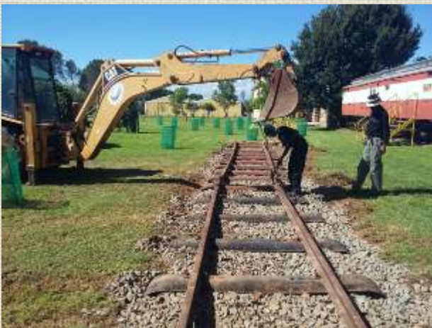
The final alignment was done with the help of the TLB.
