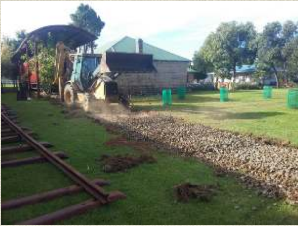
Our Track bed was ready and the 2 panels were fitted.
