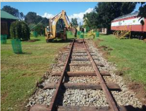
The final alignment was done with the help of the TLB.
