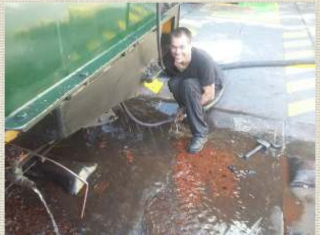
Below left: Washing out from the smoke box end towards the foundation ring where we could Remove all the scale and sludge from the boiler.
