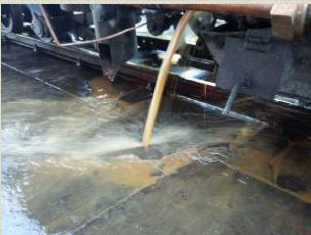
Below: Dissolved scale was washed out of the boiler.
