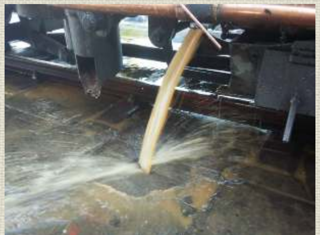
Below: Dissolved scale was washed out of the boiler.
