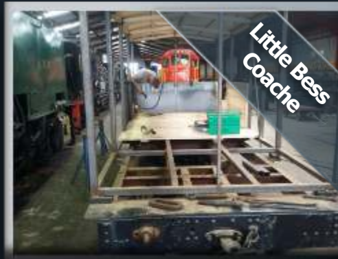
Steam Shed Upgrade
