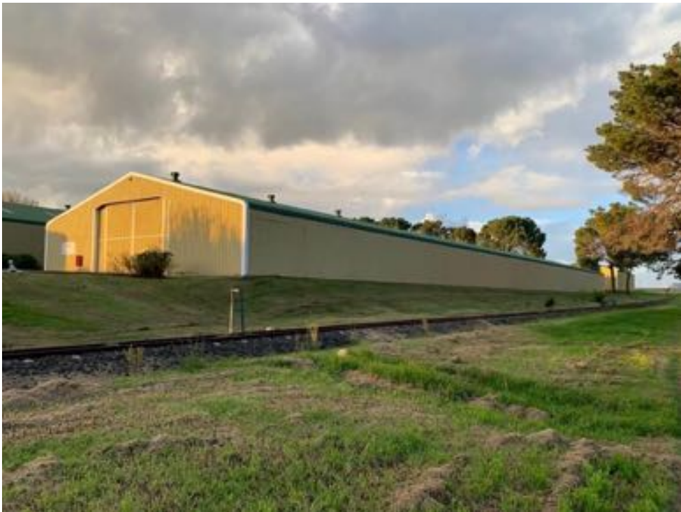
The railway Carriage and Wagon Shed.
