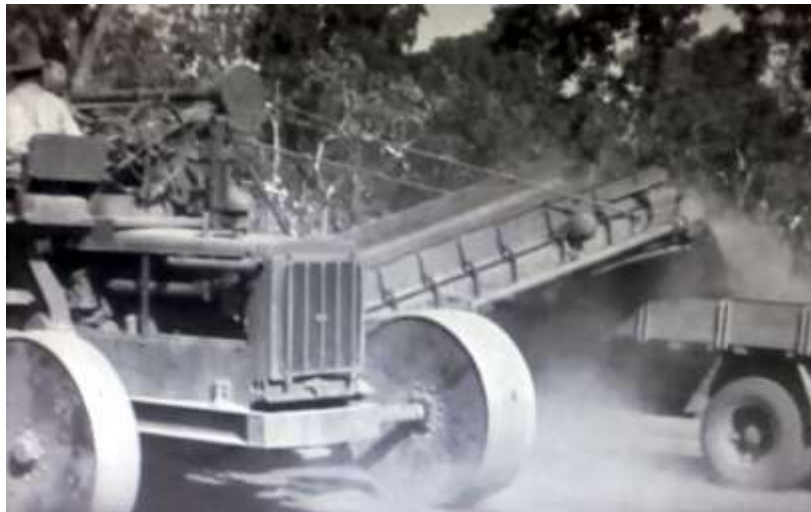
The other side of the elevator had a large plough disc cutting the base trench. They could be used to move the soil to crown the road centre or fill the trucks as seen above and on the left.
