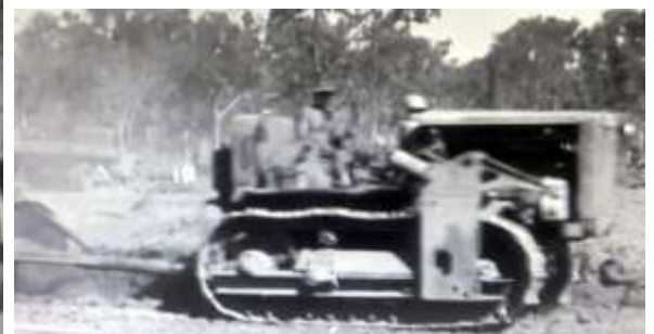
The other side of the elevator had a large plough disc cutting the base trench. They could be used to move the soil to crown the road centre or fill the trucks as seen above and on the left.
