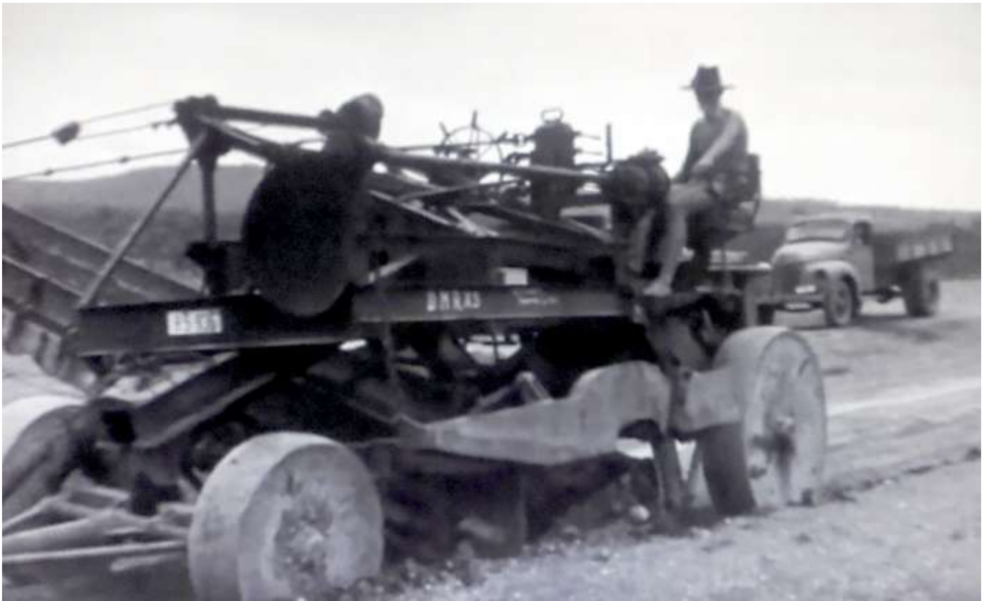
The other side of the elevator had a large plough disc cutting the base trench. They could be used to move the soil to crown the road centre or fill the trucks as seen above and on the left.
