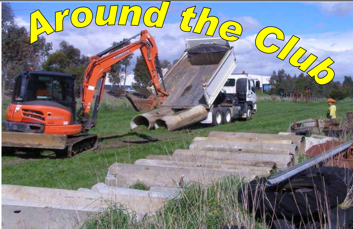
The pipes being unloaded along the East boundary
