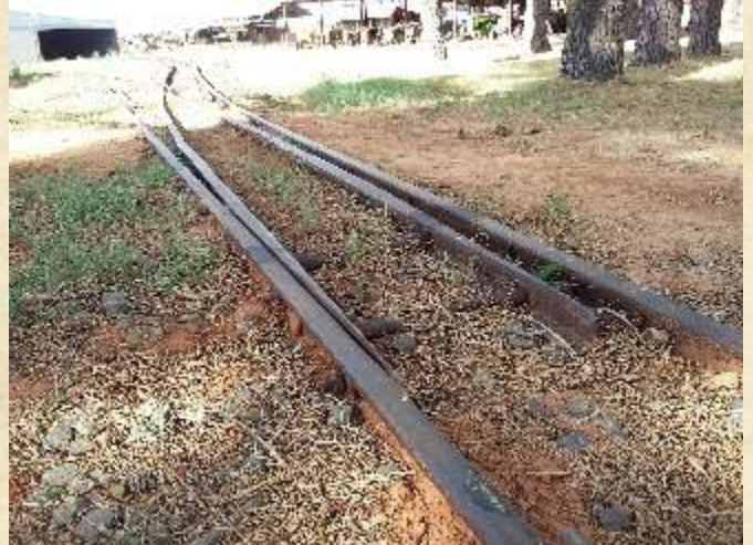
Below Right: No tumbler and points need lifting.
