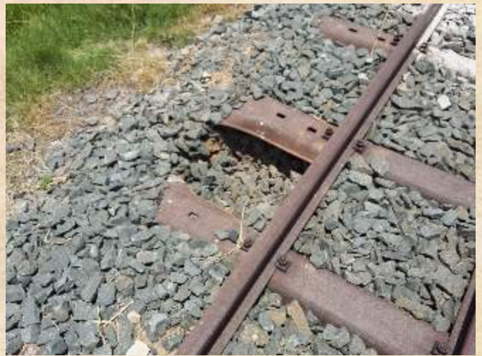
Below right: Culvert collapsing on the section Vailima Hult to Pandora junction.
