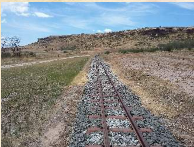
Below Left: Screening needed on curve just before Pandora Junction.
