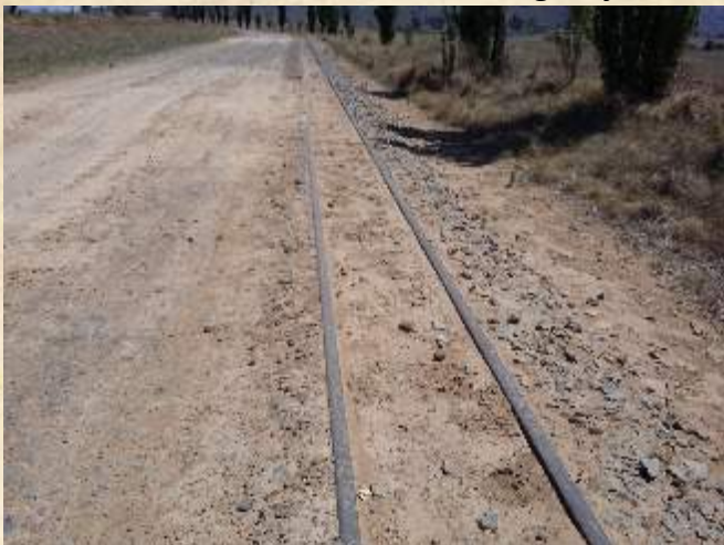
Section Hoekfontein to Grootdraai urgently needs screening.
