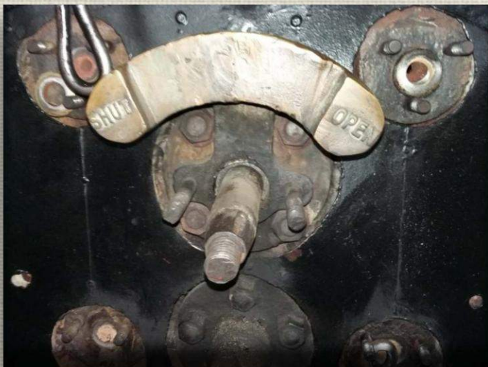
Below Left: The regulator gland removed. The old asbestos rope will be removed And repacked with new asbestos rope.
