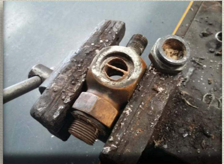
Below: Test cork being stripped and asbestos removed.
