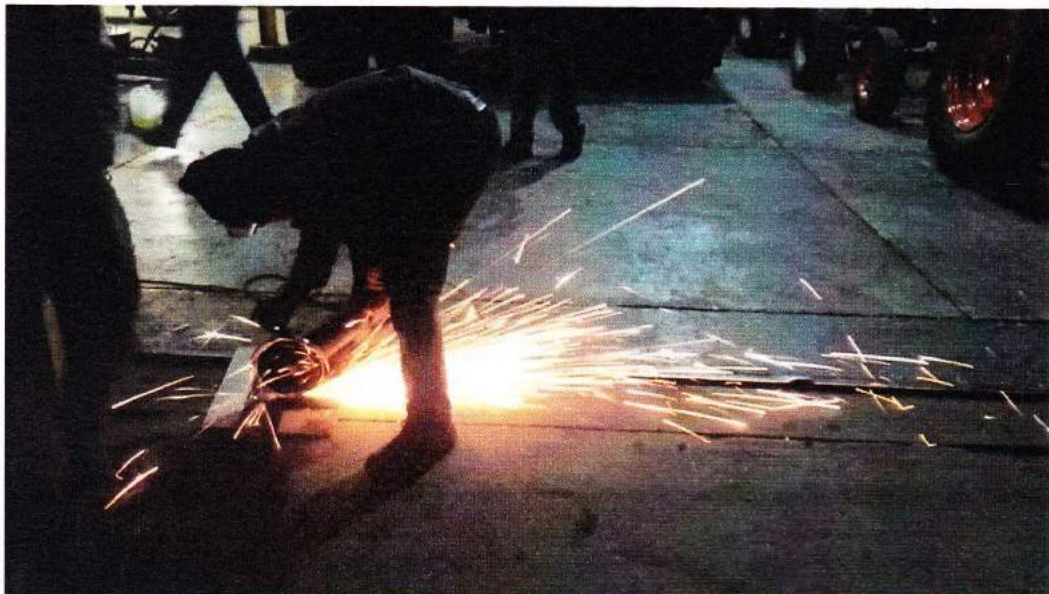
Figure 5: Late night repairs
