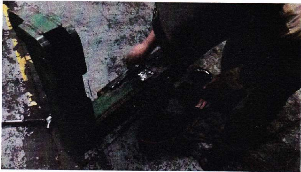
Figure 8: Emergency repairs underway
