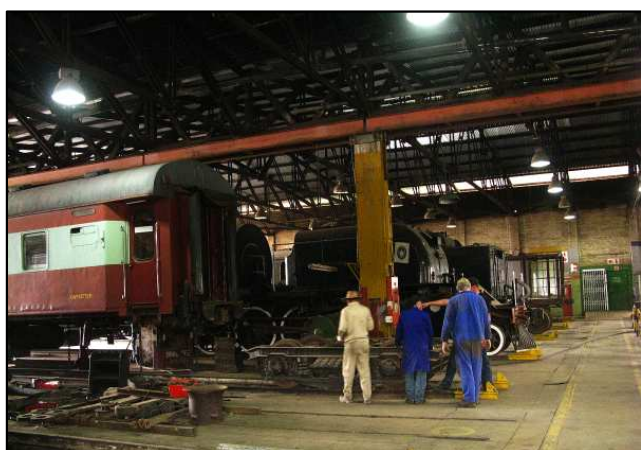
P21 - Coach lifting is underway on one of the Sandstone Day sitters. The old fashioned bar frame bogie had already been withdrawn from under the jacked-up and was undergoing inspection, lubrication and service.
