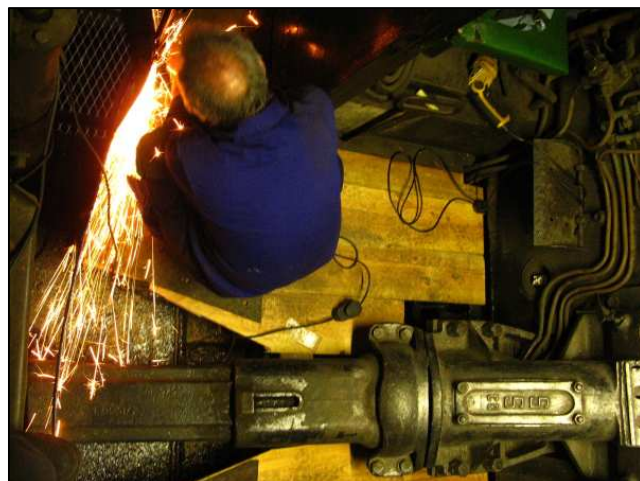
P08 - The entire cab floor was stripped and re-laid from aircraft packing timbers. (!) It wasn't part of the contract, but the cab floor was too rotted to be safe. Gordon is seen grinding down the old welds on the toe plate and the nosing caps before the tread plates could be reinstalled.
