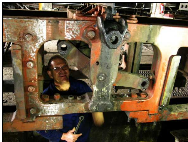
P26 - The inter-axle equaliser links were all removed with the aim of cleaning, inspection and rebushing if necessary.
