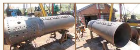
The boiler barrel fitted to firebox end. All the doubler plates have been riveted into the outer firebox wrapper and the stay holes drilled. The boiler barrel has been drilled, reamed and bolted ready for riveting and caulking.
