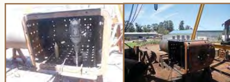
Drilling through the foundation ring into the outer firebox wrapper. The outer wrapper riveted up to the throat plate and backhead.
