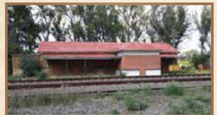
Sannaspos Station today, somewhat derelict, but intact.
