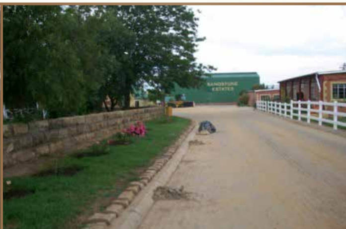
The sandstone edging along the main entrance road has been repaired.
