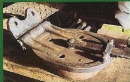
The firehole door was removed in order to re-align it.
