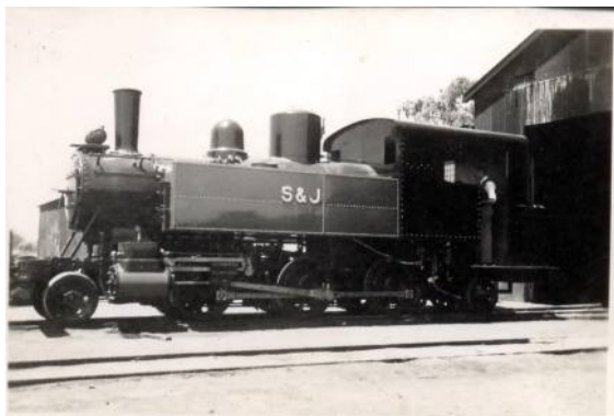
The Porter after an extensive rebuild in 1949
