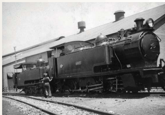
Eskom Komati 0-8-0, 1926 Ex Witbank Pwer Station. 1948. Photo: Dave Parsons
