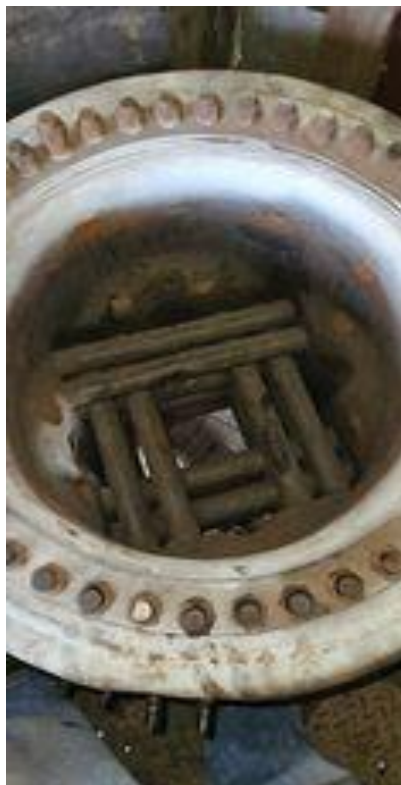
The boiler from the top after testing showing the tubes.
