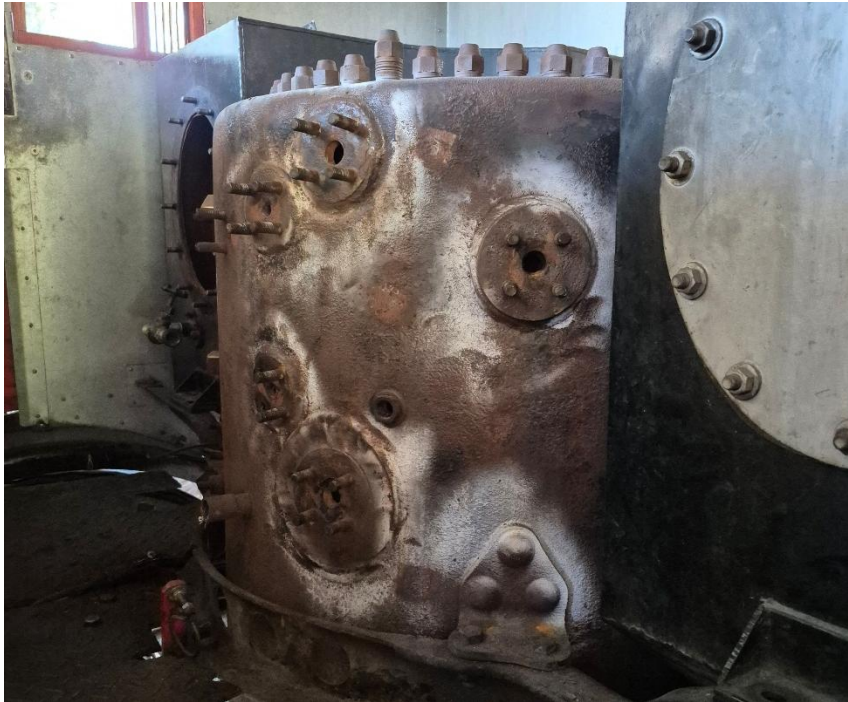
The boiler test complete
